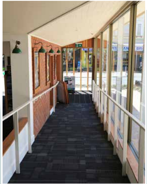
TE KUITI VISITOR INFORMATION CENTRE - ENTRANCE TO RAILWAY STATION BUILDING 1.
