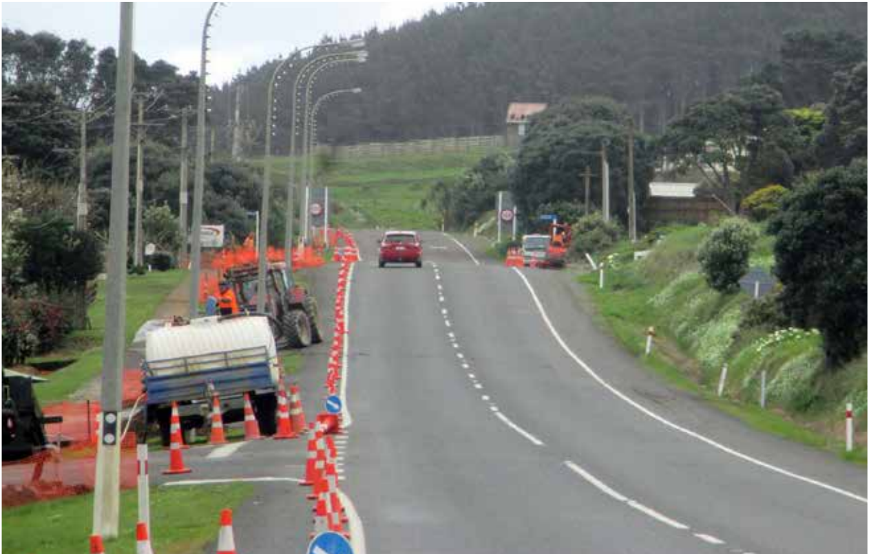
MOKAU WATER RETICULATION - MAIN PIPE REPLACEMENT PROJECT
