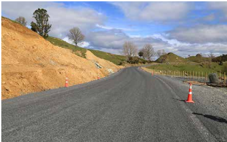
REHABILITATION OF KUMARA ROAD
