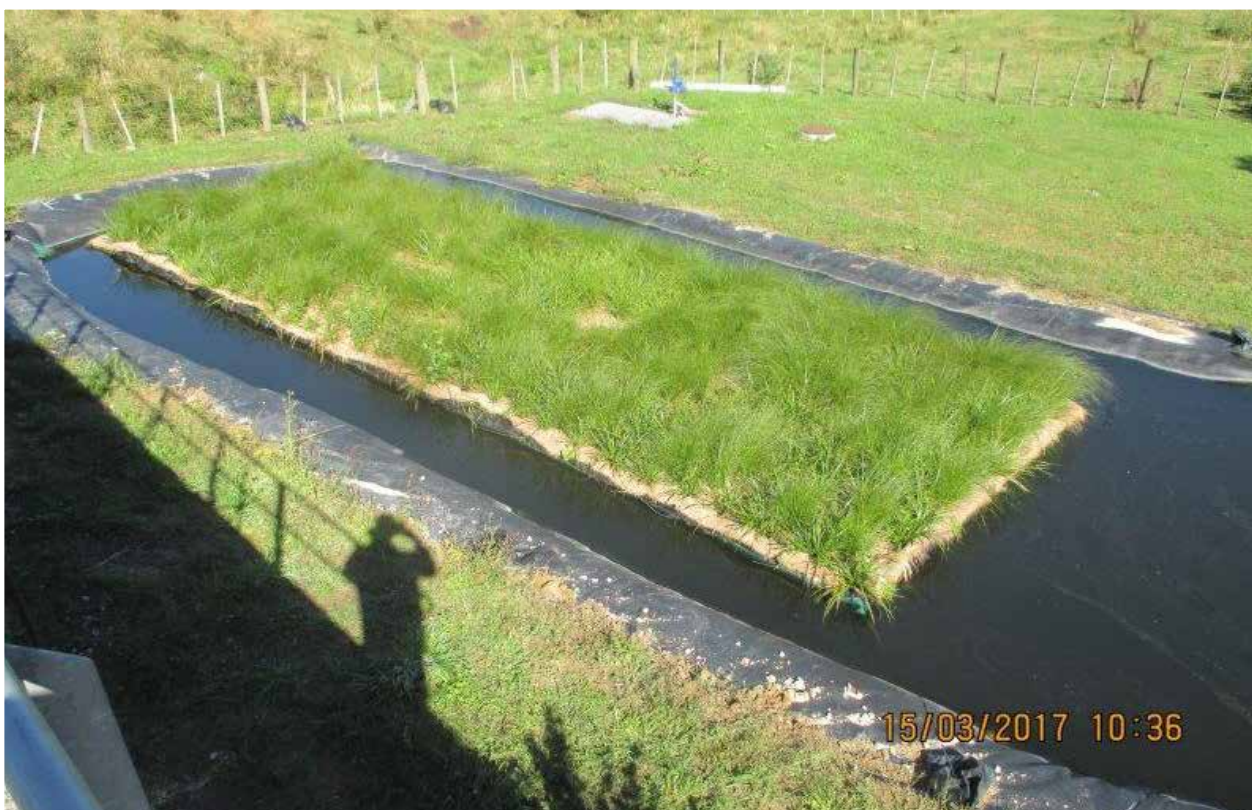
BENNEYDALE WASTE WATER TREATMENT PLANT
