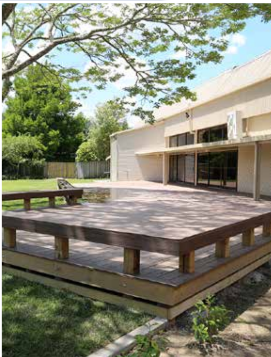
THE NEW DECK AREA AT THE LES MUNRO CENTRE
